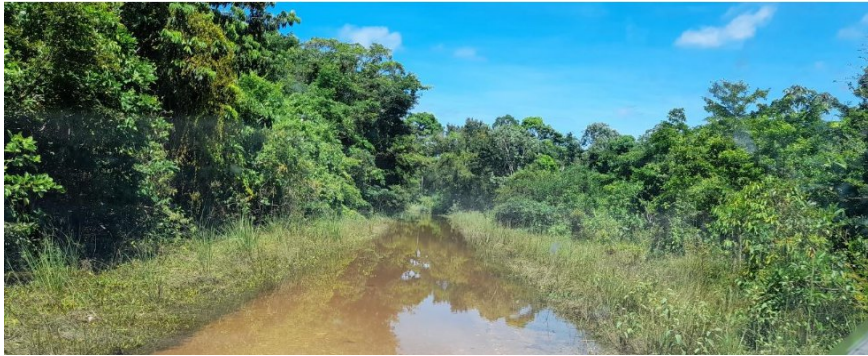
Figure 27: Boom Creek Road during flooding (Source: Boom Creek Village Needs and Assets Assessment, 2021).
