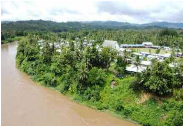
Figure 10 Upper Wainimala River: Serea Village which is experiencing riverbank erosion affecting houses close to riverbank
