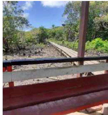
Figure 14 Timber support struts built by youth of Tavuya village to access the village during high tide to ensure safety and allow for free movement during flooding
