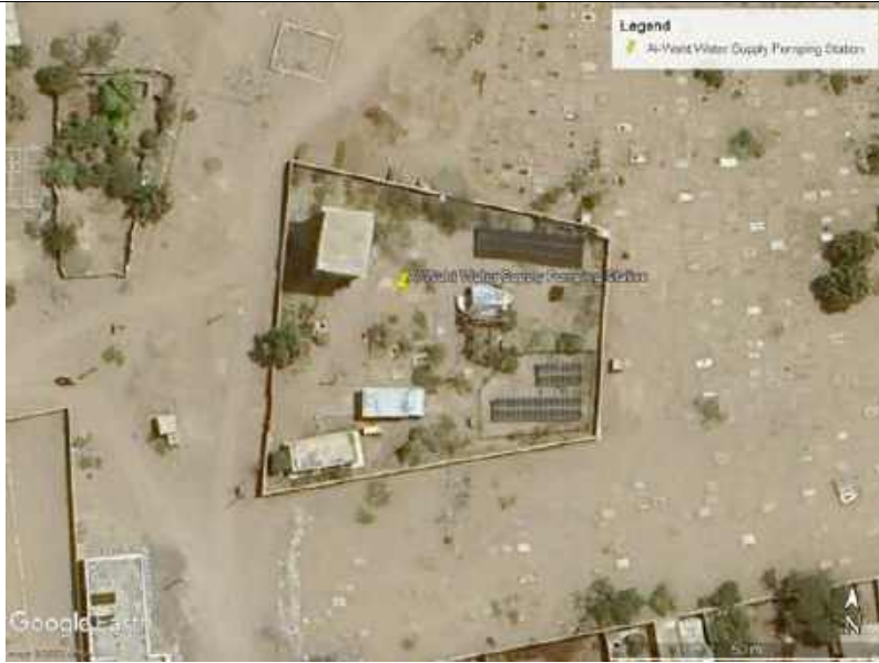
Figure 14-15. Al-Waht City and Location of Water Supply Pumping Station
