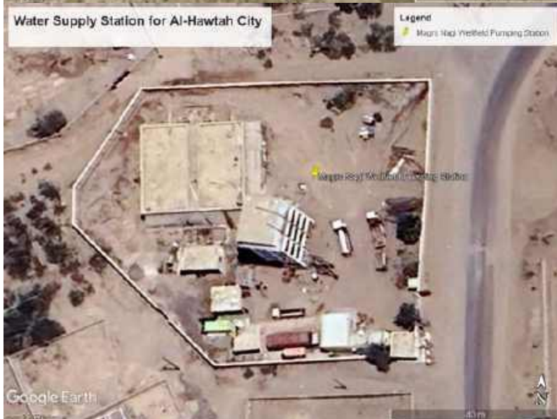
Figure 16-17. Al-Hawtah City and Water Supply Pumping Station
