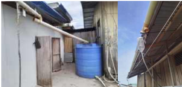
Figure 5. Existing rainwater harvesting systems, Sitangkai
