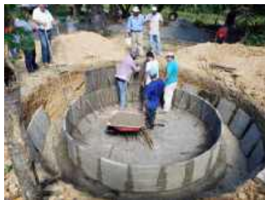
FIGURE 10. EXAMPLE OF 16-THOUSAND-LITER PLATE TANK
