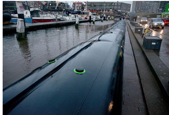
The Netherlands – Urban Area Supported by Water Authority
