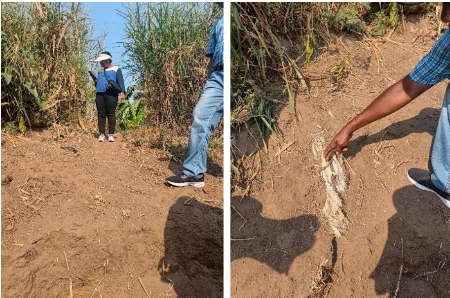
Erosion of the Kochi river banks due to high flow velocities
