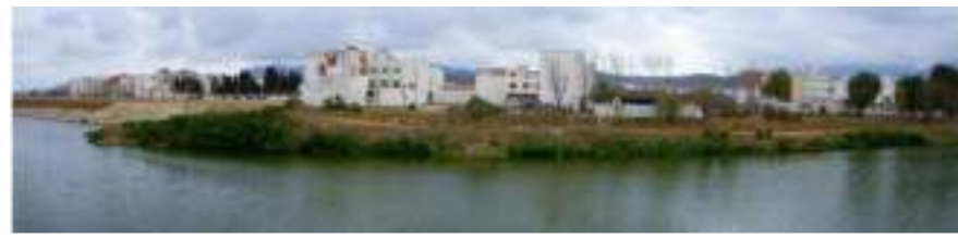
Fig 4. Area at risk of flooding in the Municipality of Tetouan (Coelma neighborhood)
