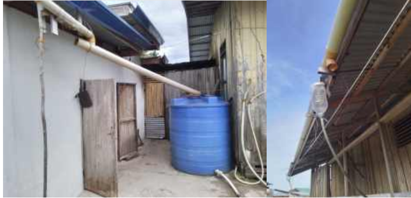
Figure 5. Existing rainwater harvesting systems, Sitangkai
