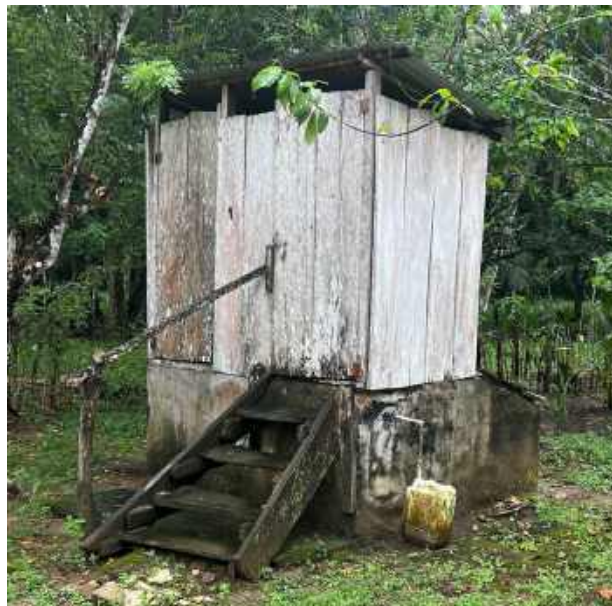
Figure 30: Boom Creek Sustainable Harvest International Latrine (Source: Site visit, 2023).
