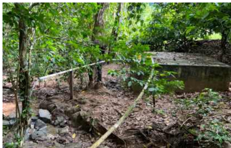
Figure 34: Spring Water Reservoirs with PVC Pipes to the Village (Source: Site visit 2023).
