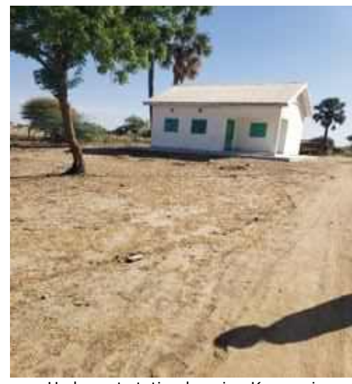
Hydromet station housing Kousseri
