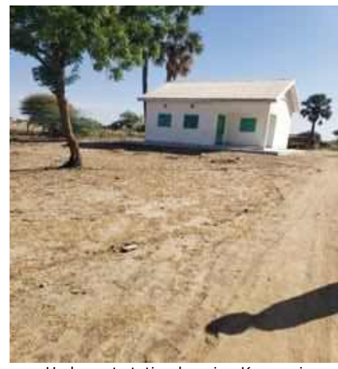
Hydromet station housing Kousseri
