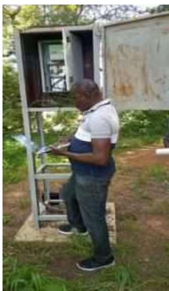
Hydromet Station (CHAD)
