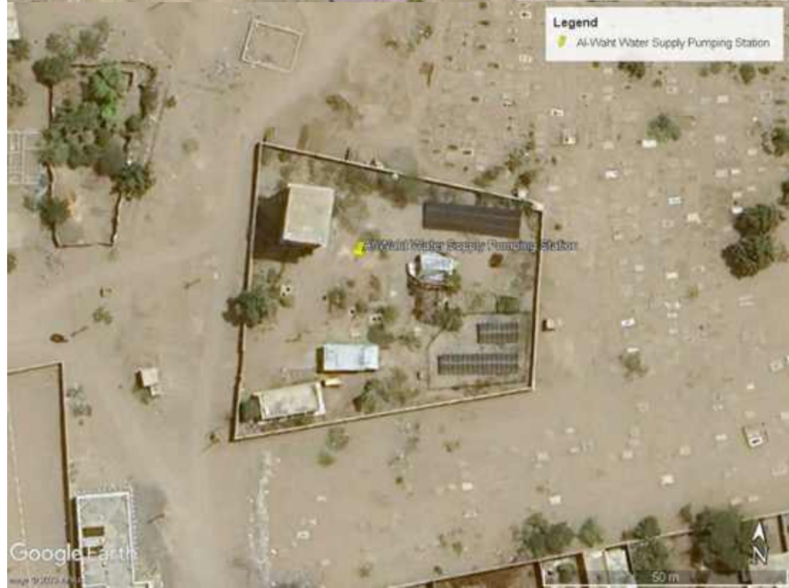
Figure 61 Al-Hawtah city and water supply pumping station
