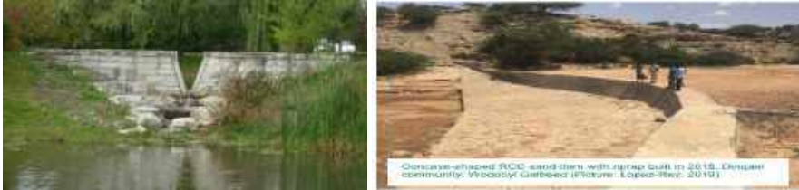
Figure 3: V-Shaped/Notched Weirs 34 (Left) and Sand dam (Right) 35
