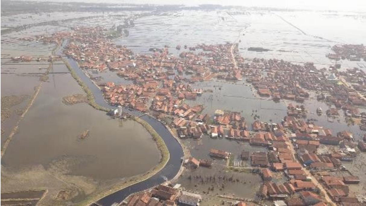
Figure 4. Severe Flooding in Pekalongan City
