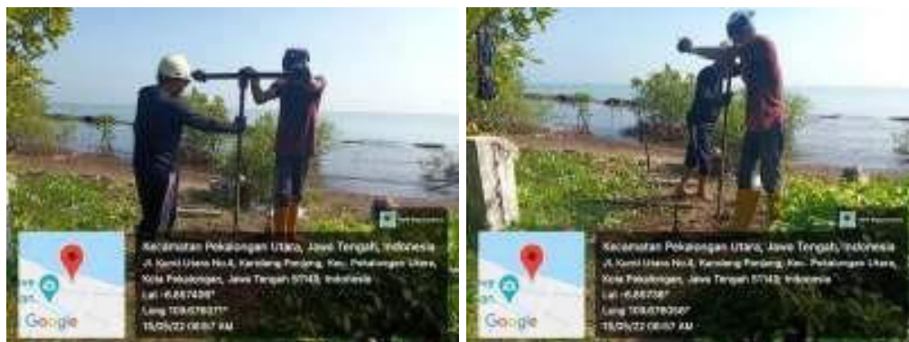
5.1.1.64 Figure 6.5 Boring process
