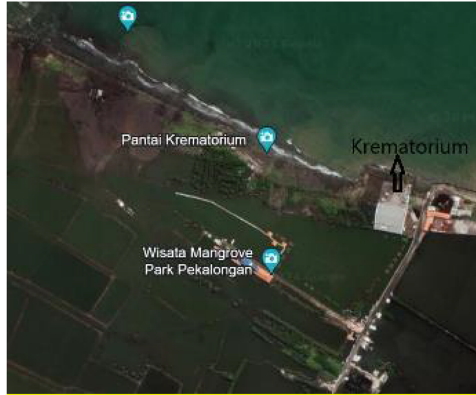
Figure 13 Bird view of the breakwater construction site in front of “Pantai Krematorium”
