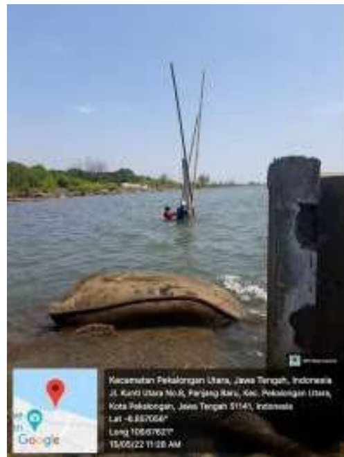
Installing a Tide Staff
