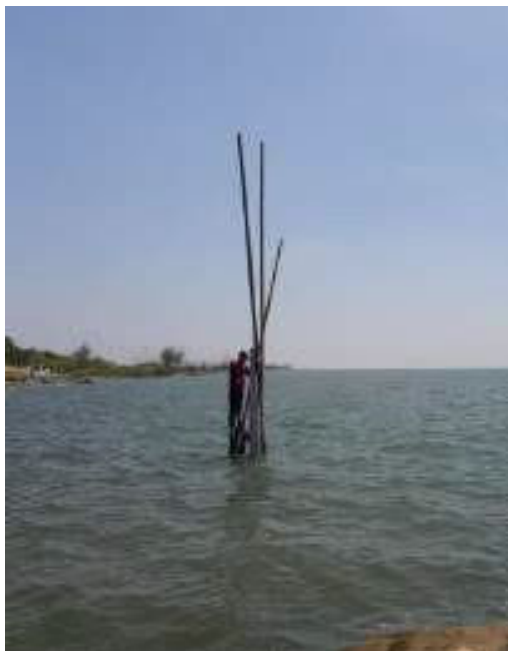
Installing a Tide Staff
