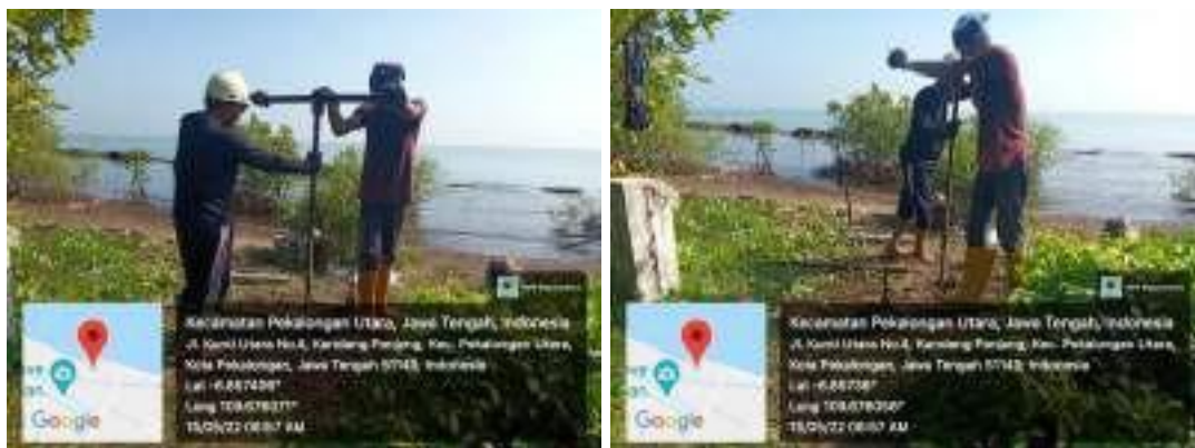
5.1.1.64 Figure 6.5 Boring process
