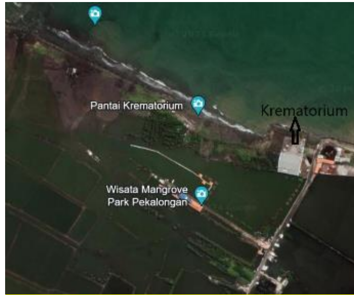
Figure 13 Bird view of the breakwater construction site in front of “Pantai Krematorium”
