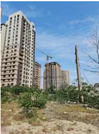
Figure 37: Tall residential apartment blocks are being built along the abandoned rail tracks
