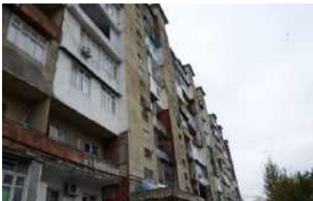
Figure 27: A.2-1: Typical multi-story building in Nefchala without access to water during drought (source: Anar Valiyev)
