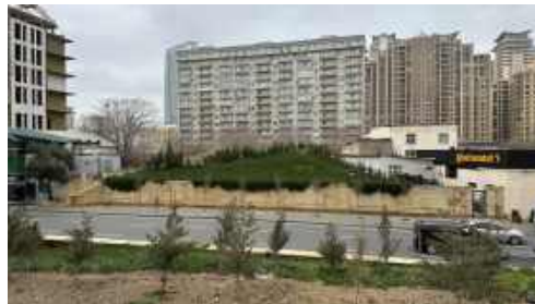
Figure 25: A.1-5: Road cutting across the former railway corridor, limiting accessibility to "green corridor"
