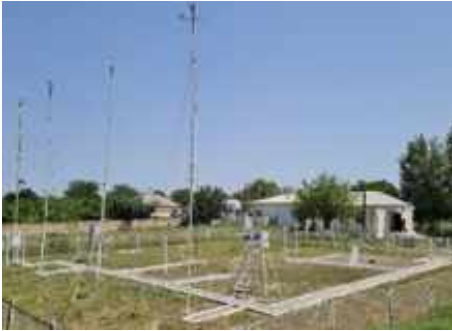
Figure 44: Meteorological Station in Neftchala district.
