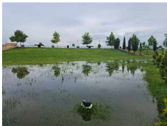
Figure 46: Vast areas of the public park realized along the Caspian Sea in Astara City may remain waterlogged for weeks after the seasonal rains in spring, but risk becoming scorched earth during the hot summer months because of the lack of water.
