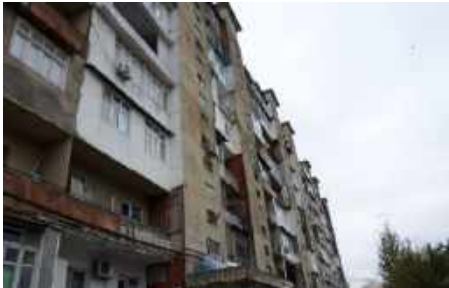
Figure 27: A.2-1: Typical multi-story building in Nefchala without access to water during drought (source: Anar Valiyev)
