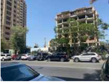
Figure 21: A.1-1: Housing under construction in Baku city centre
