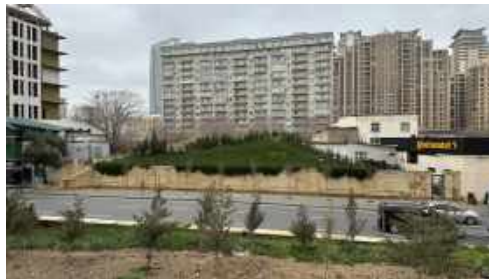
Figure 25: A.1-5: Road cutting across the former railway corridor, limiting accessibility to "green corridor"
