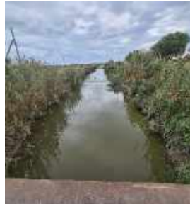
Figure 28: A.2-2: Irrigation canal washing salinity from agricultural fields into the Kura River catchment area (source: Anar Valiyev)
