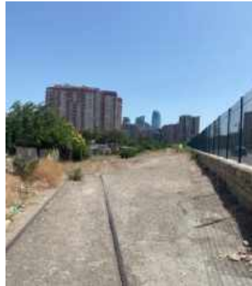
Figure 24: A.1-4: Cement coverage along the former railway line
