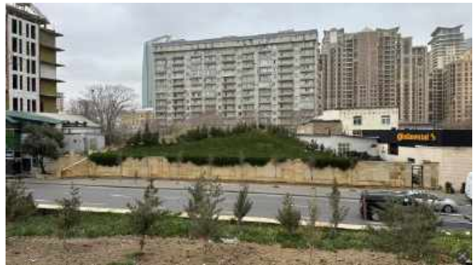
Figure 25: A.1-5: Road cutting across the former railway corridor, limiting accessibility to "green corridor"
