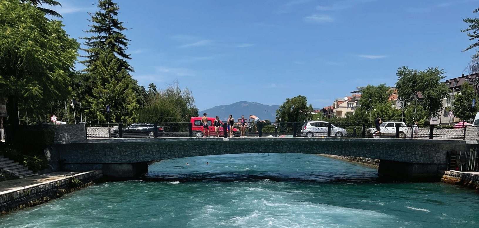
Removing deposited sediment and overgrown vegetation from the river led to resilient flood risk planning in the Black Drin River, Struga, North Macedonia Photo by UNDP Euroasia
