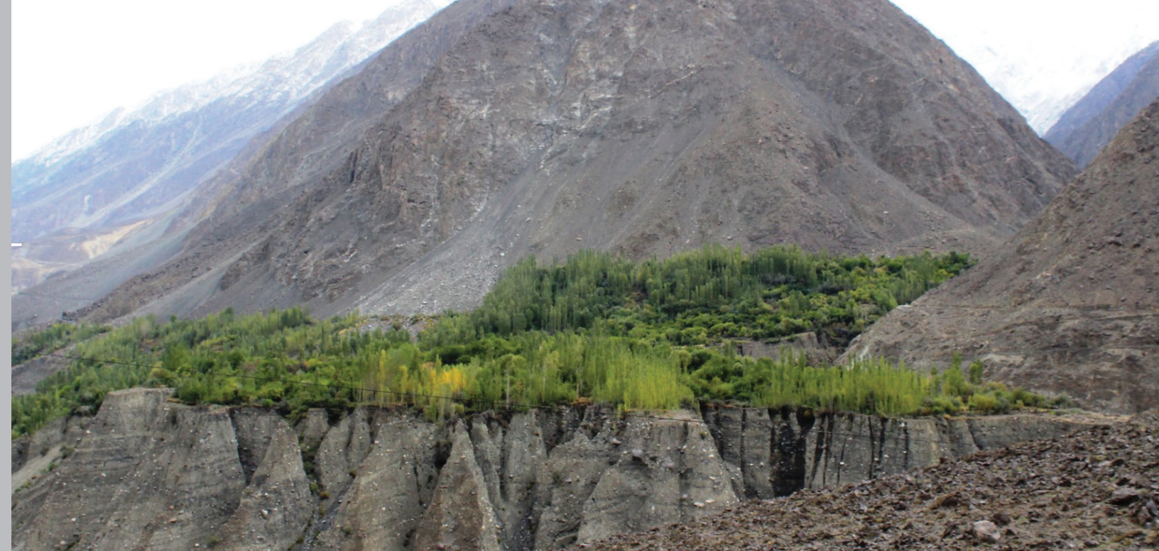
Gabion wall built by local communities to effectively control flash flood, project funded by AF in Northern Pakistan. Photo by UNDP
