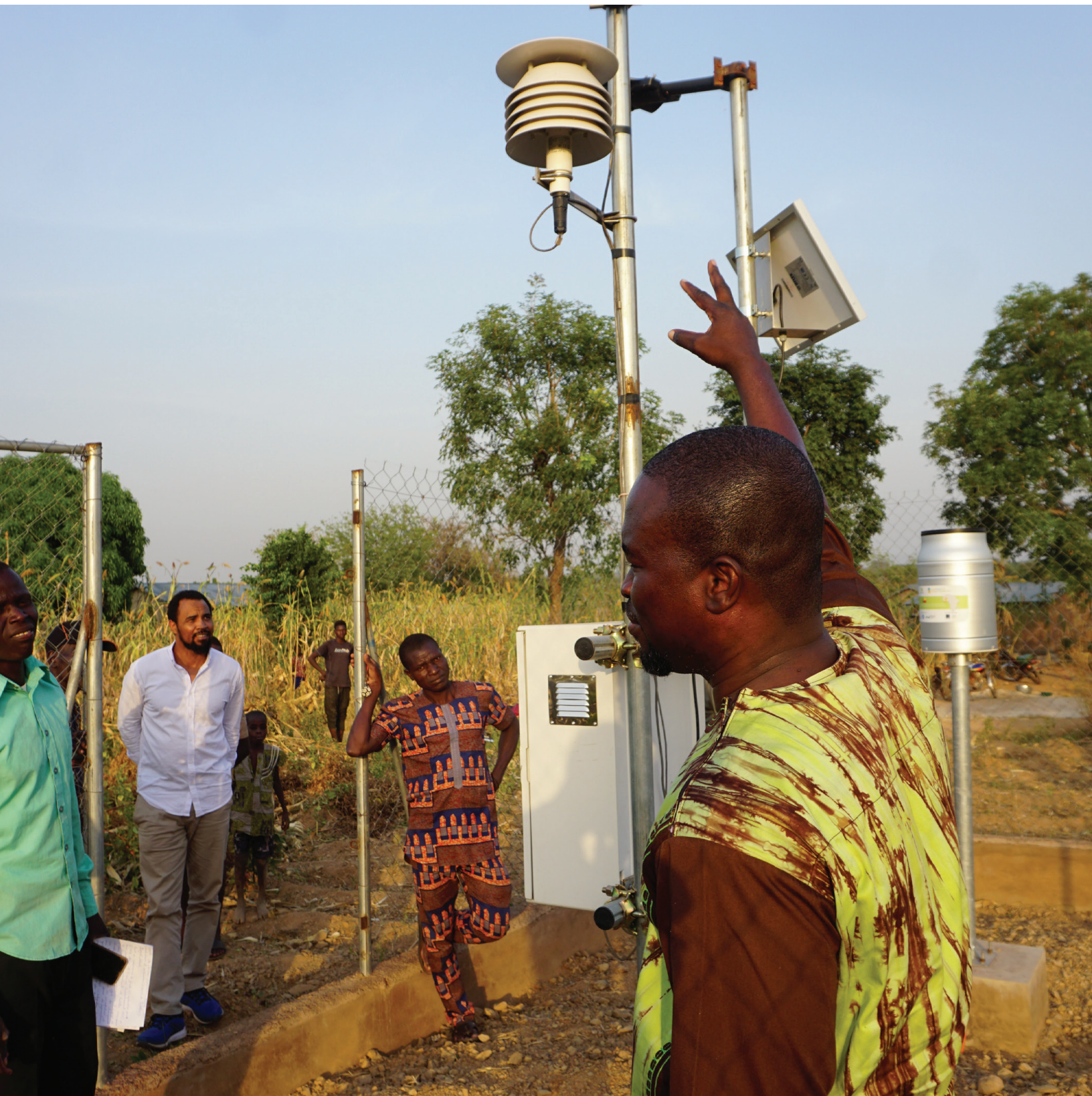
Automatic weather stations installed in the West Africa, Volta Basin - Benin, Cote D'Ivoire and Ghana Photo by Adaptation Fund
