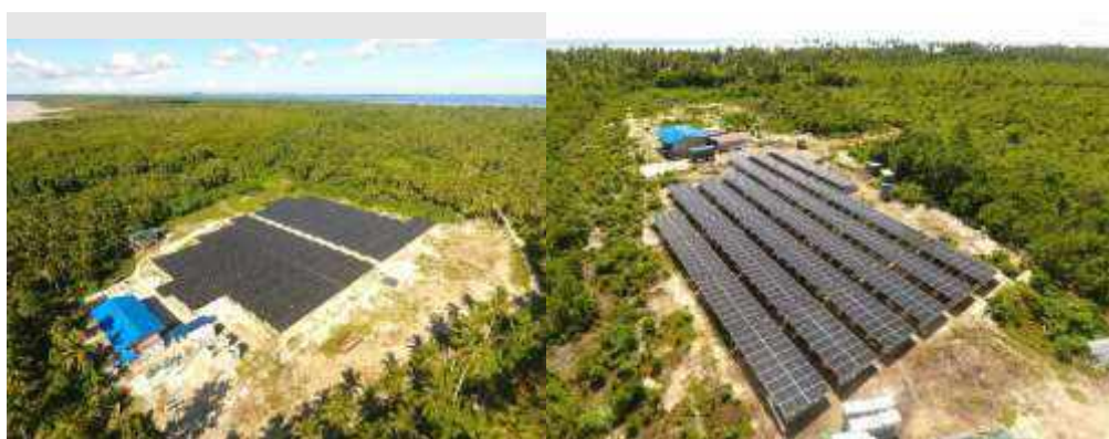
Figure 14. Photovoltaic plants and diesel generators deployed by the RETS project in Sibutu and Sitangkai, as of October 2021. Source: The RETS project
