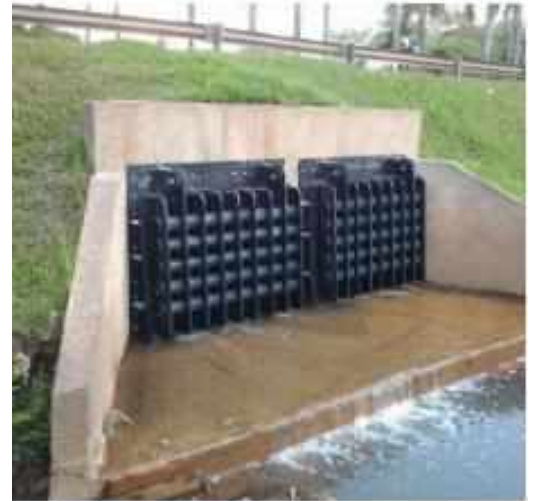
Figure 2 – Example of Flap Gate - FLOGATE HDPE, link
