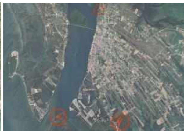
Figure 3 – Wastewater management interventions in Koh Kong Province
