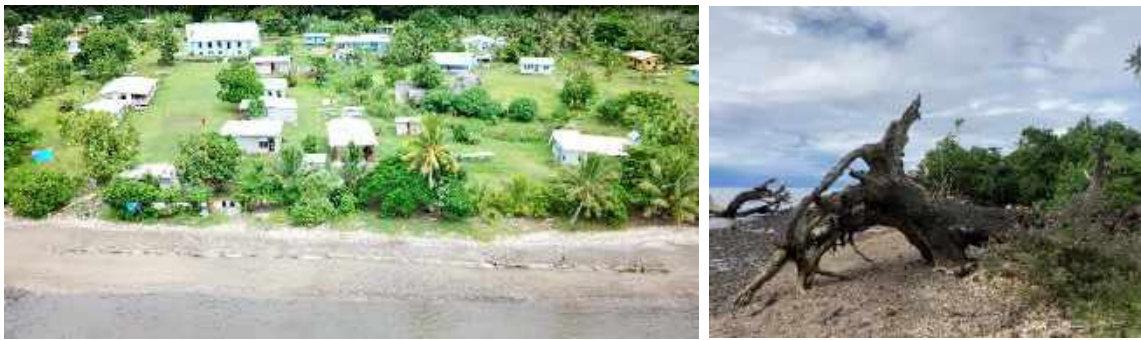
Figure 45: Site for NbS seawall installation in Nabuna Village.
