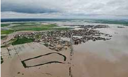
Figure 3: Flood in Golestan Province 2019
