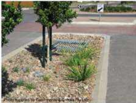
Figure 55: Component of a drainage system
