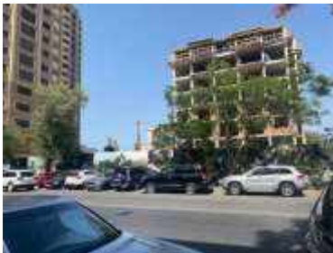
Image A.1-1: Housing under construction in Baku city center
