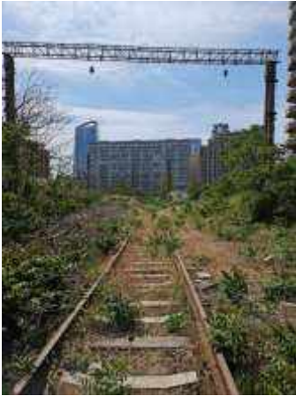
Figure 27: In the background, an older and rundown residential block, visible also in the bird's eye view below (*).
