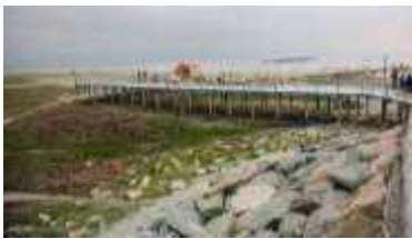
Image I.4-3: Seawater retreat in Bandar-e-Torkaman
