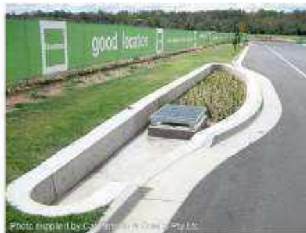
Figure 54: Component of a drainage system
