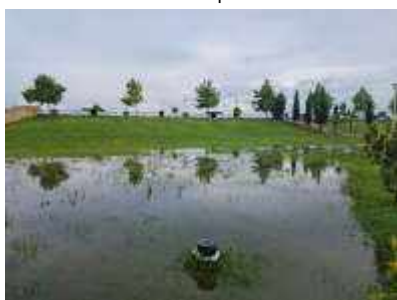
Figure 34: Vast areas of the public park realized along the Caspian Sea in Astara City may remain water logged for weeks after the seasonal rains in spring, but risk becoming scorched earth during the hot summer months because of the lack of water.
