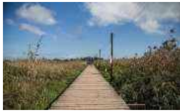
Image I.2-4: Wooden Bridge in Bandar-e-Kishahr
