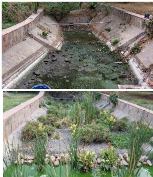
Figure 10 – Outfalls Conversion of a drainage canal into a subsurface flow constructed wetland
