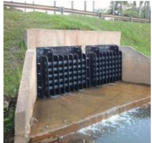
Figure 2 – Example of Flap Gate - FLOGATE HDPE, link
