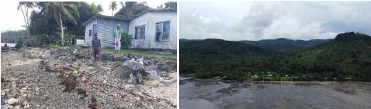
Figure 30: Project site at Sese Village
