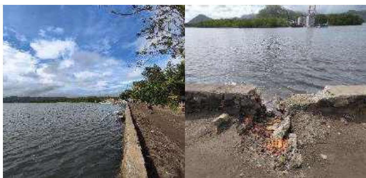
Figure 7 Existing condition of embankments in South Lembar village
