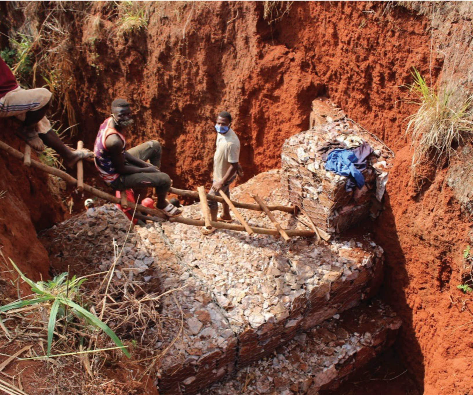
Gully rehabilitation in the Republic of Rwanda, as part of a five-country regional AF-funded project. Photo by ACC-LVB Project Coordination Team
