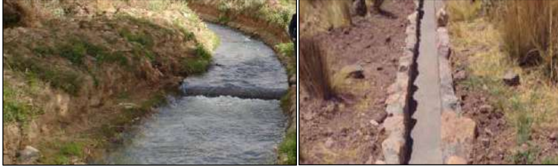
FIGURE 5. UNLINED IRRIGATION CANALS IN FIAMBALÁ, PROVINCE OF CATAMARCA. EXAMPLE OF A STONE-LINED CANAL, JUJUY PROVINCE
