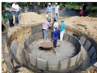
FIGURE 10. EXAMPLE OF 16-THOUSAND-LITER PLATE TANK
