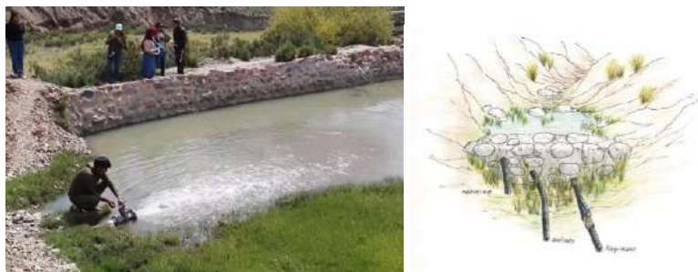
FIGURE 3. STONE RETAINING WALL OF THE MINI DAMS
