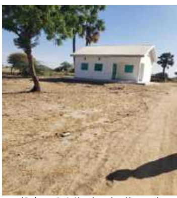
Hydromet station housing Kousseri
