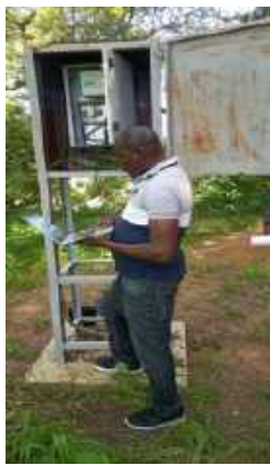
Hydromet Station (CHAD)
