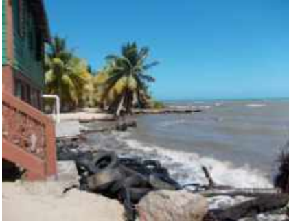
Figure 9: Image depicting erosion in Dangriga (NCCO, 2019)
