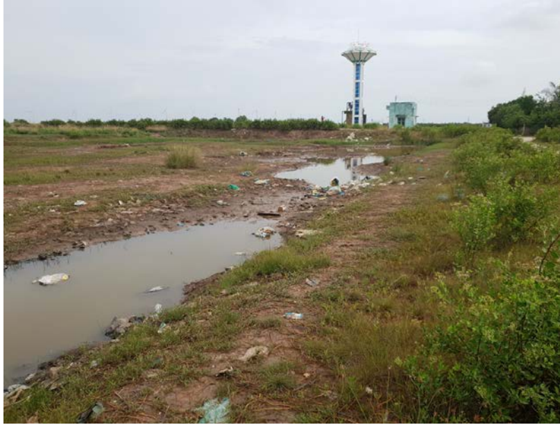
Figure 11. Water tank in the community
