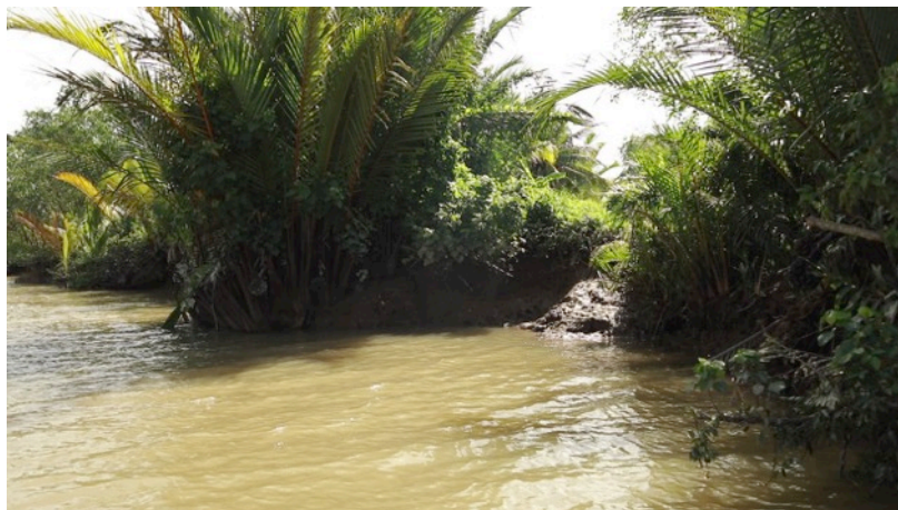
Figure 12. Rive bank erosion
