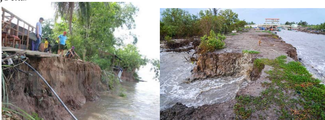
Figure 2. The images of land erosion in the Mekong Delta
