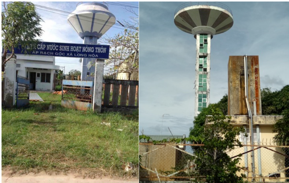
Figure 7. Water tank and treatment system in Hoa Minh and Long Hai
