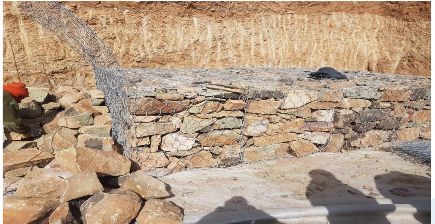
Perimeter protection structure
