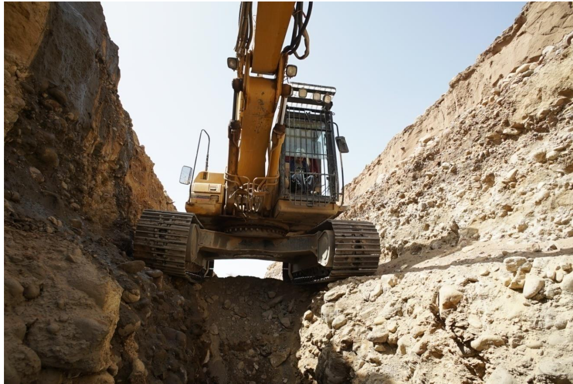
Rehabilitation works of a khetara
