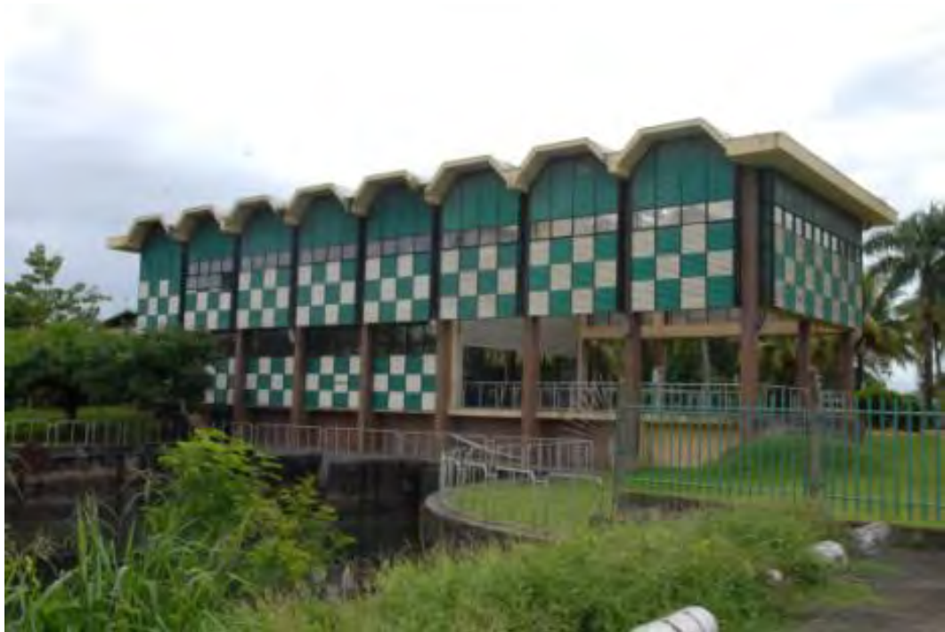
Figure 3-7: Existing Pump House
