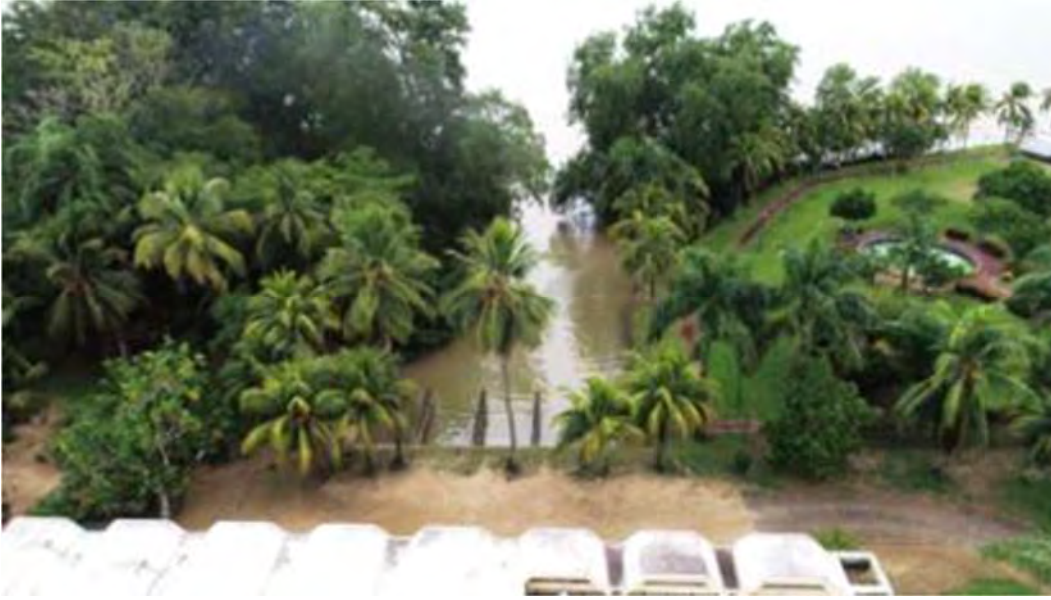
Figure 37: Existing Condition of Outflow Area
