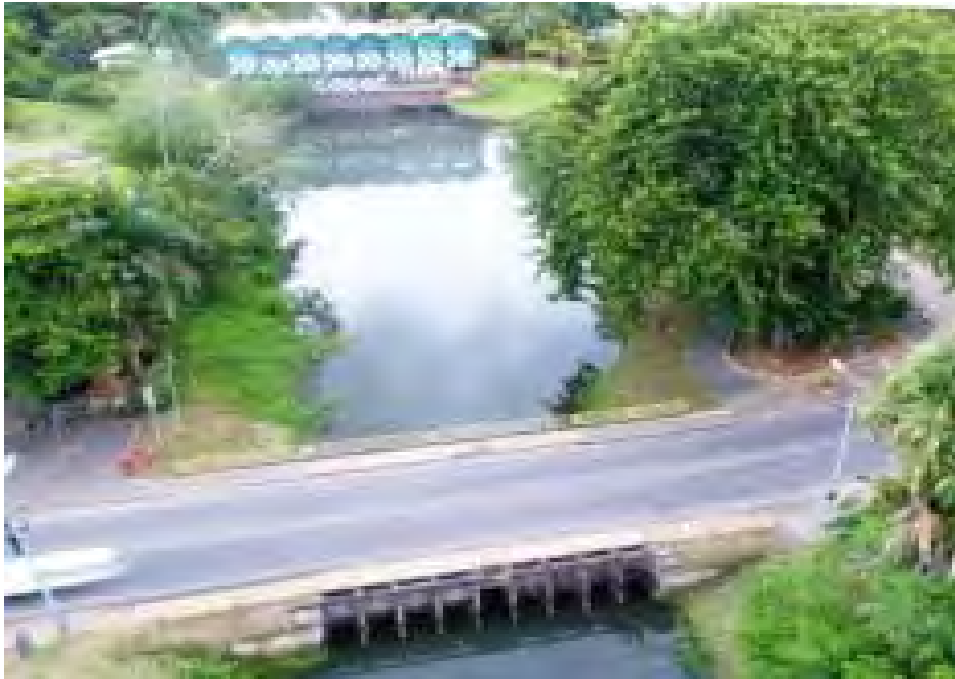
Figure 35: Existing Condition of Water Basin
