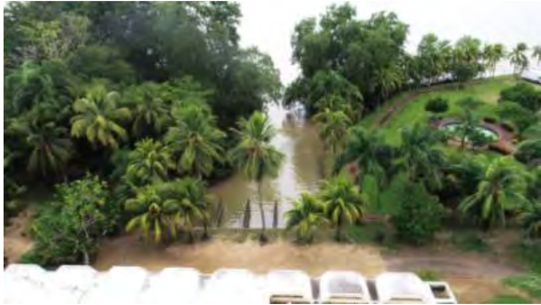
Figure 3-8: Existing Condition of Outflow Area
