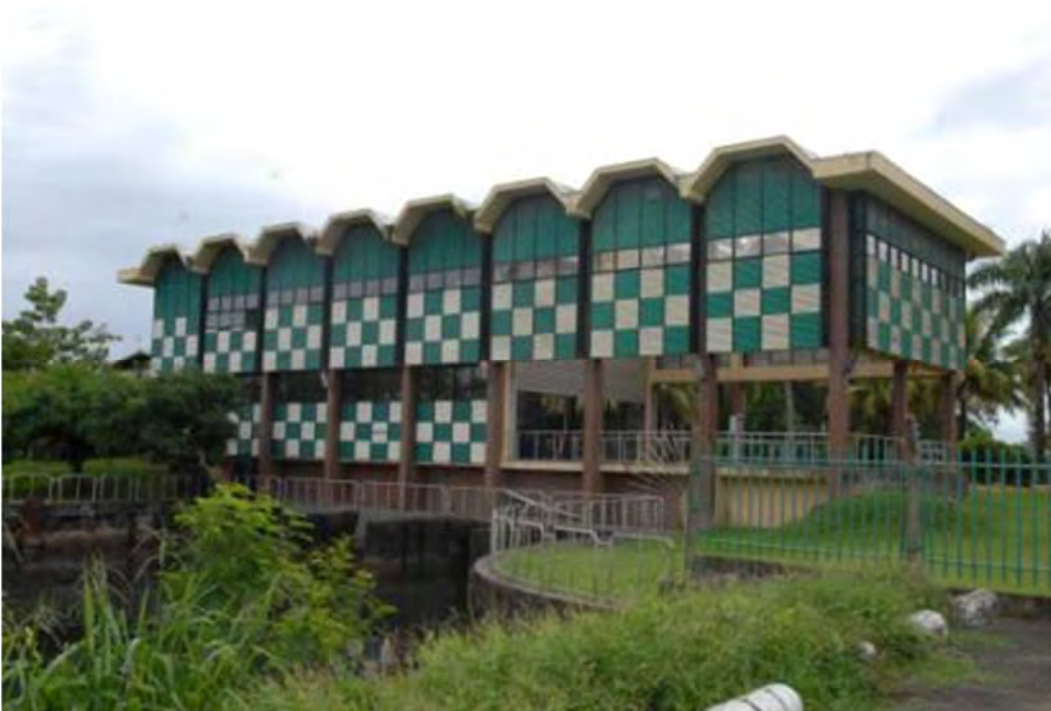
Figure 36: Existing Pump House
