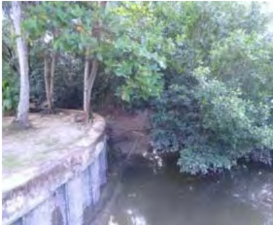
Image16: Sheet piles of steel
