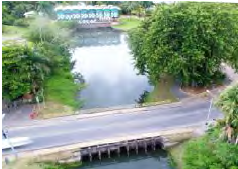
Figure 3-6: Existing Condition of Water Basin
