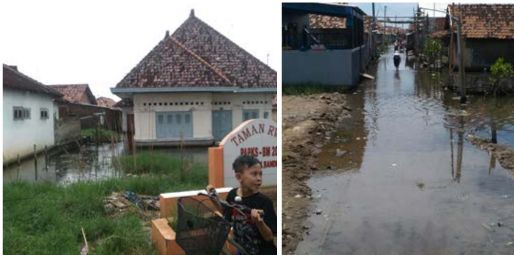
Figure 7. Inundated Settlement Area in Pekalongan Utara (before Rainfall) (Site Observation, 2017)
