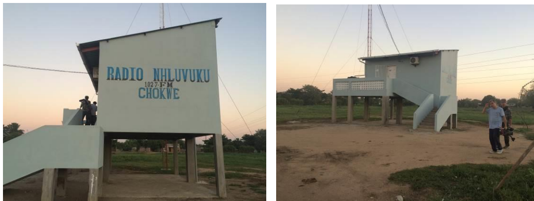
Figures 37 and 38: Elevated radio station built by UN-Habitat after the 2013 floods, so that it can continue functioning and alerting the local population in case of major floods
