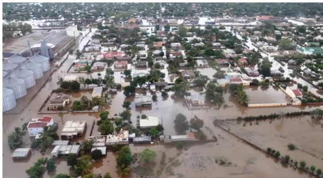
Figures 29 and 30: Chokwe floods, January 2013
