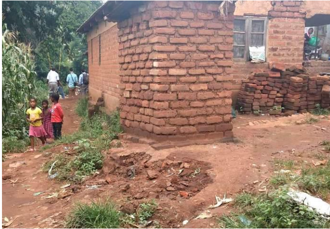
Figure 26: Typical housing construction standards in Zomba
