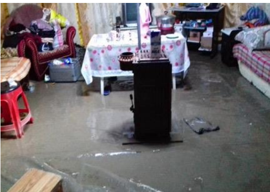
Basement of the 12 th apartment of Khilchin hothon – flood water and ground-water penetrating from the walls and floors leading to power cut restriction of 670 households Photo (UN-Habitat June 2017)
