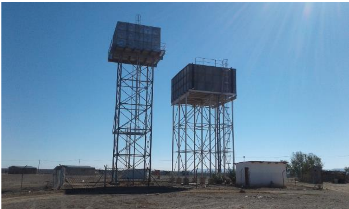
Figure 4: Water tank at Bethanie
