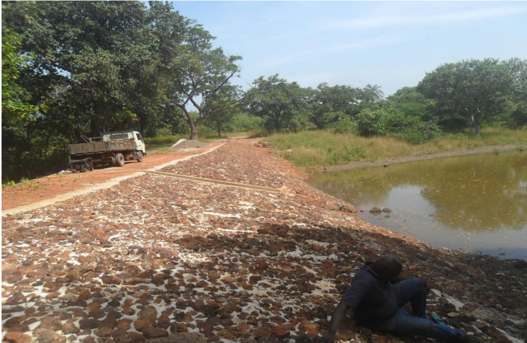
Partial view of micro dam (with a downstream water drainage channel) built in Bajocunda at the end of 2016 to control flood and used like a bridge
