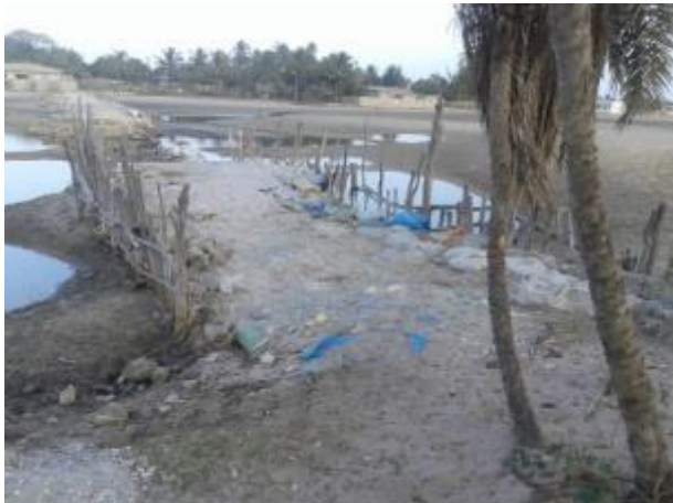
Picture 9: Ndioundiouré dike made up with shell wall, left bank
