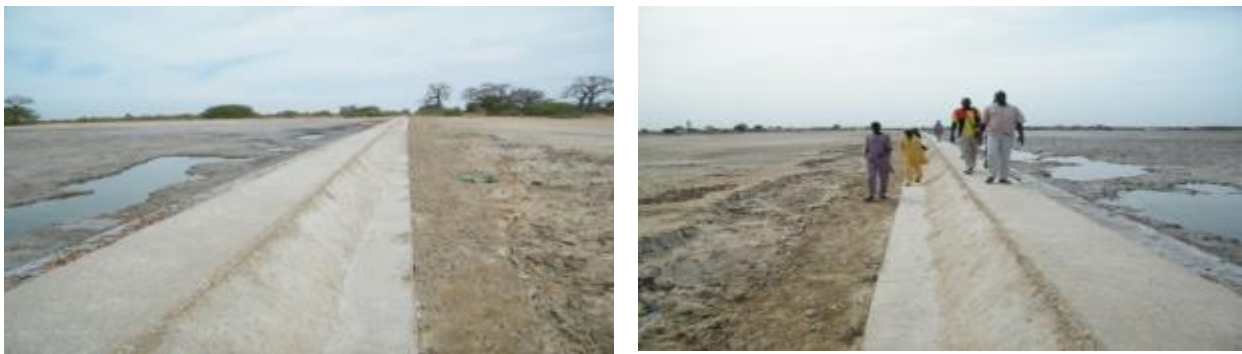
Picture 5: Compacted Earthen Dike Surfaced With Shell Concrete
