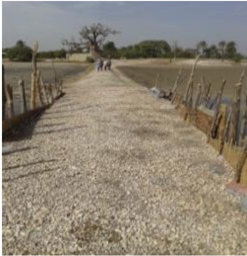
Picture 7: Ndiar dike with a shell embankment
