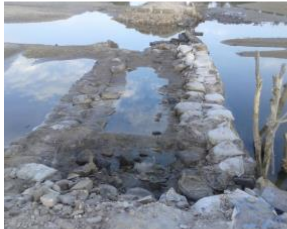
Picture 9: Ndioundiouré dike made up with shell wall, left bank
