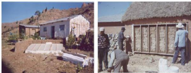
FotoPhoto: Implementation of heaters and Trombe walls, low-cost, accessible technologies.
