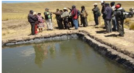
Photo: Type of earthen dyke to be constructed for the storage of snowmelt and from the short rainy season. Source: COPASA Archives (2012). The image corresponds to dykes operating in the region
