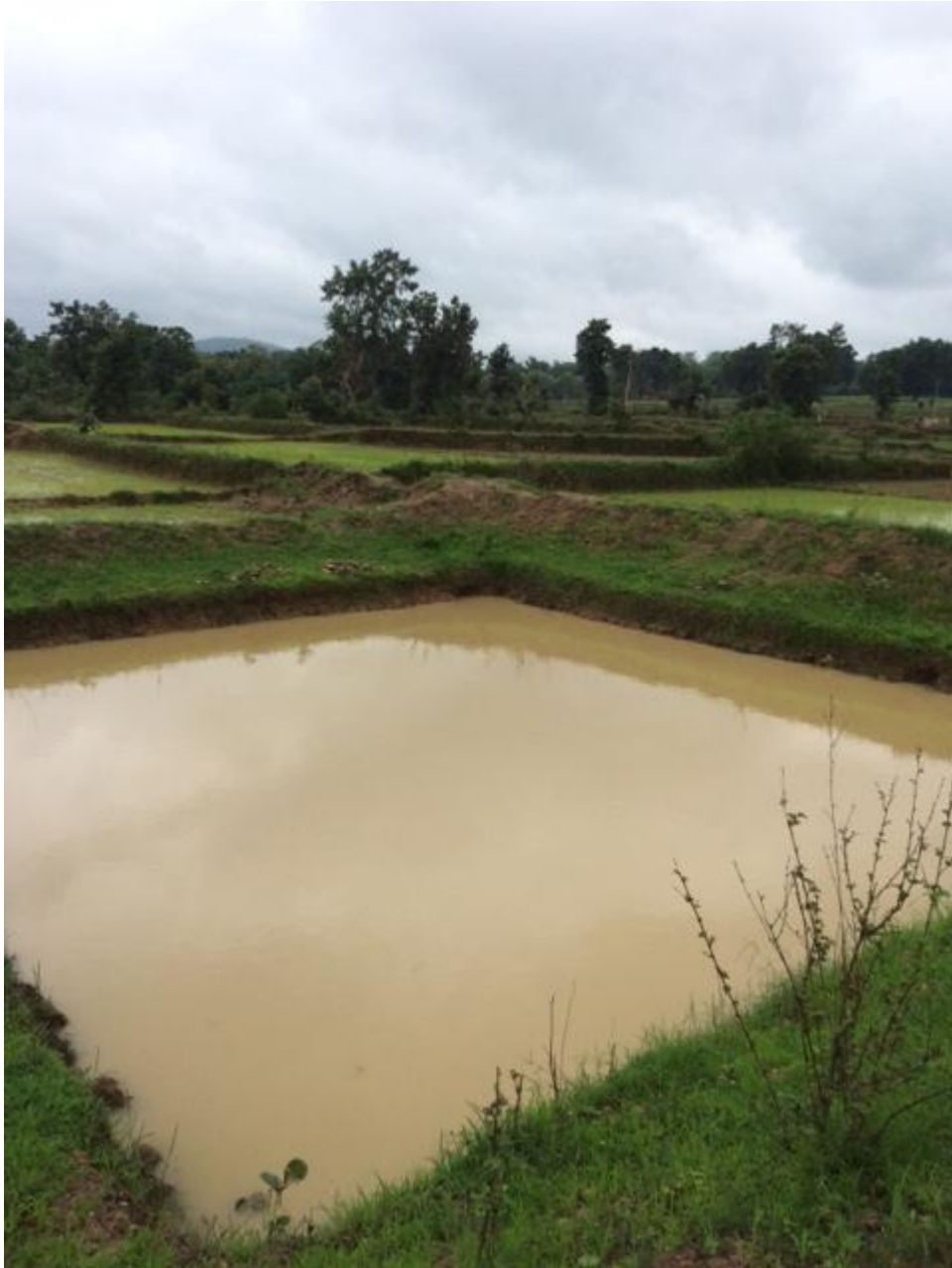
Plate 6 – A farm pond (10 meter * 10 meter * 3 meter) created in an existing project village
