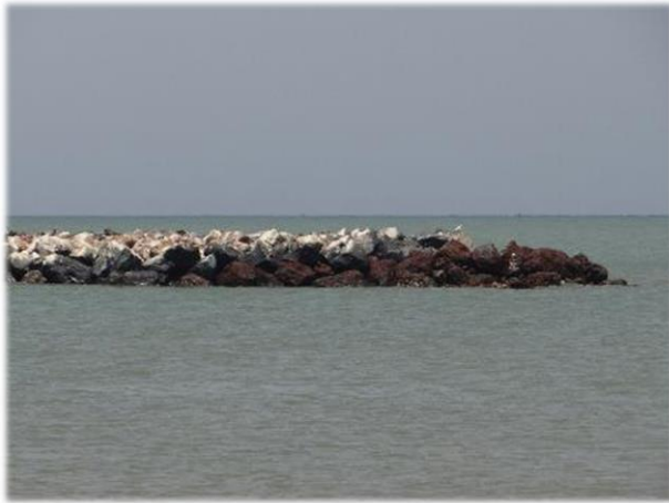
Photo 5. The extremity of one of the seawalls which contains laterite blocks on the right and basalt blocks on the left and on top.
