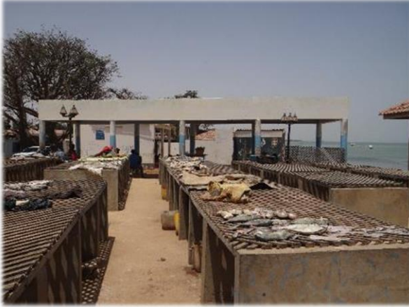
Photo 10. Drying grids and supporting structures rehabilitated by the AF-financed project.
