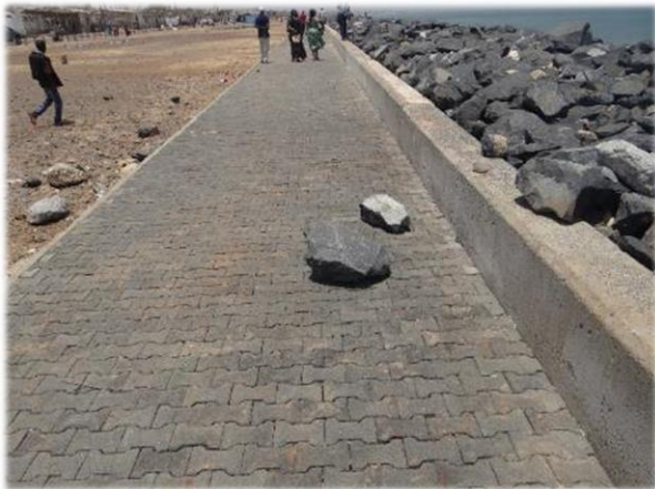
Photo 6. Basalt rocks projected onto the promenade as a result of a recent storm.
