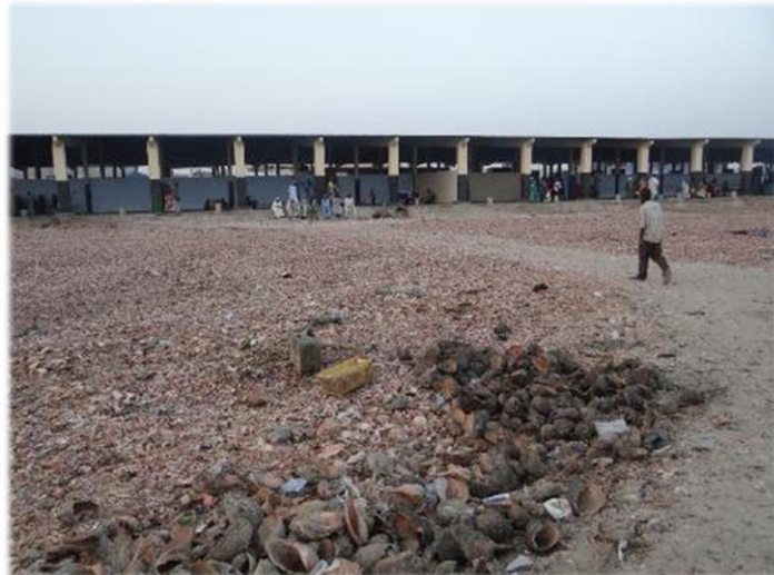
Photo 14. Artificial sand replenishment of the area between the fishing dock and the dike by means of shells and sand.
