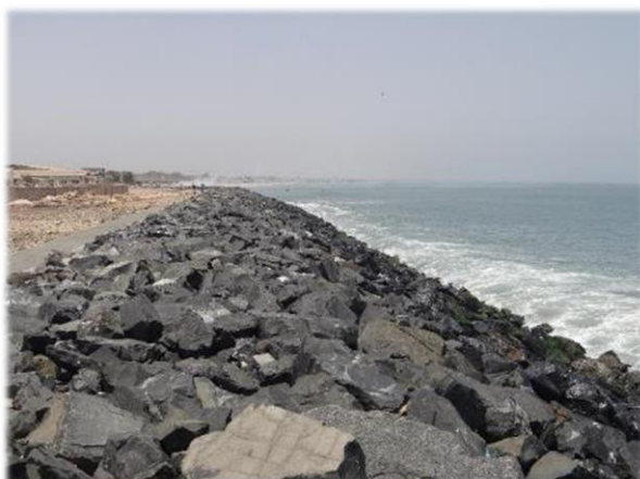
Photo 1. The basalt shell of the dike in Rufisque.
